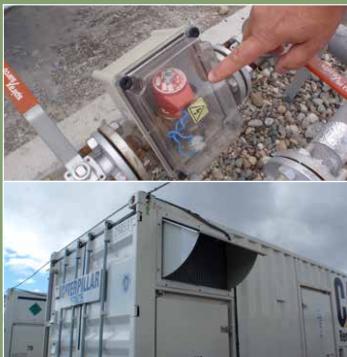
Adaptations to protect GenSet equipment in Bariloche, Argentina, from repeated airborne ash exposure following 2011-2012 eruption of Cordon Caulle volcano, Chile.
